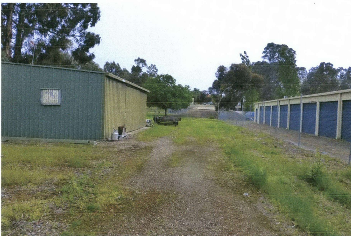
Pic 3: View looking down from the front entrance gate. There is one colour bond shed. The adjacent property to the right are storage sheds.
