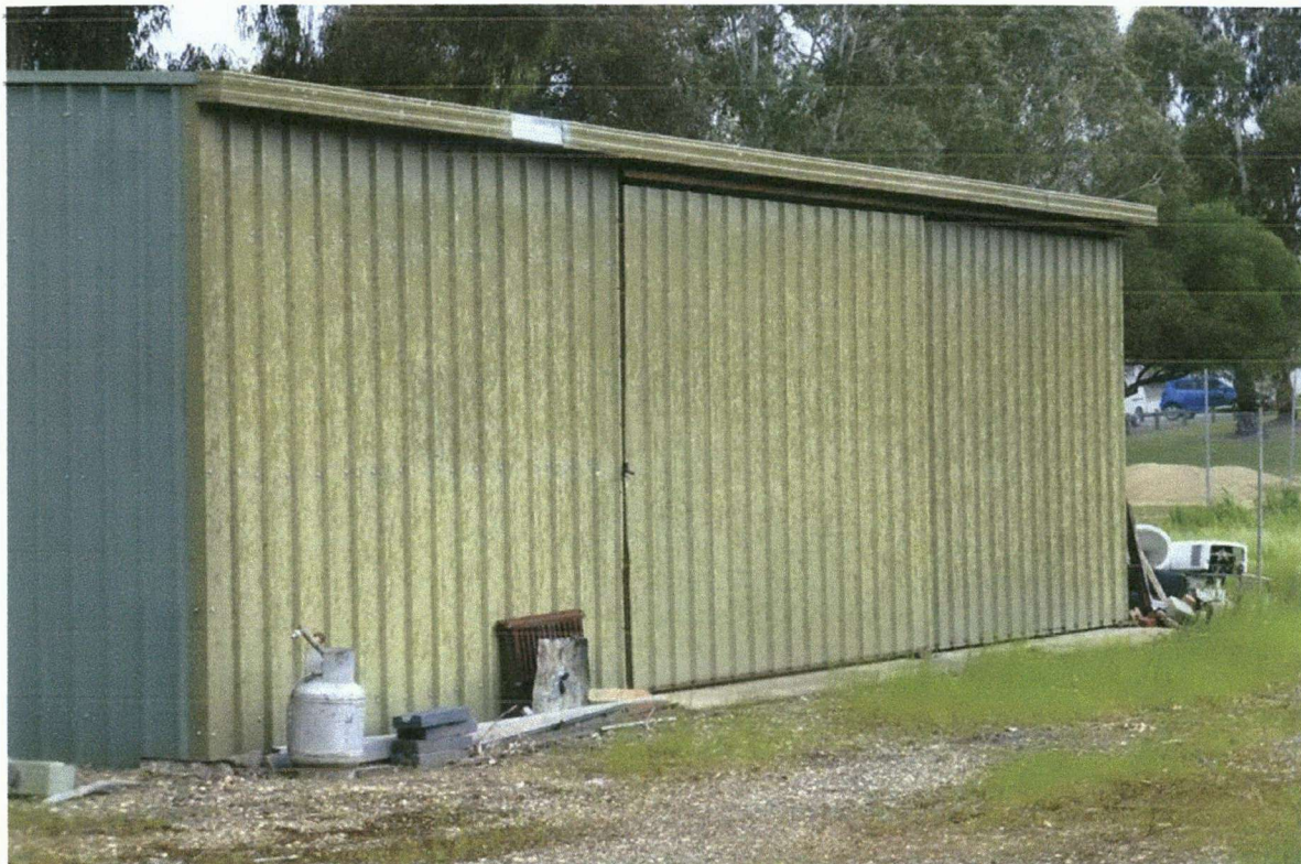
Pic 4: This is the existing colour bond shed.
