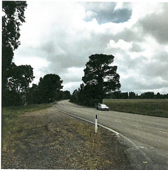
Figure 2.3: Melba Highway looking north
