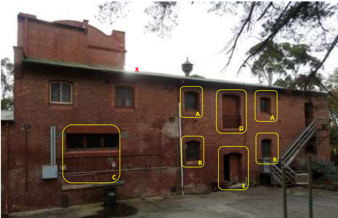
Figure 1. View of eastern wall (original building)
