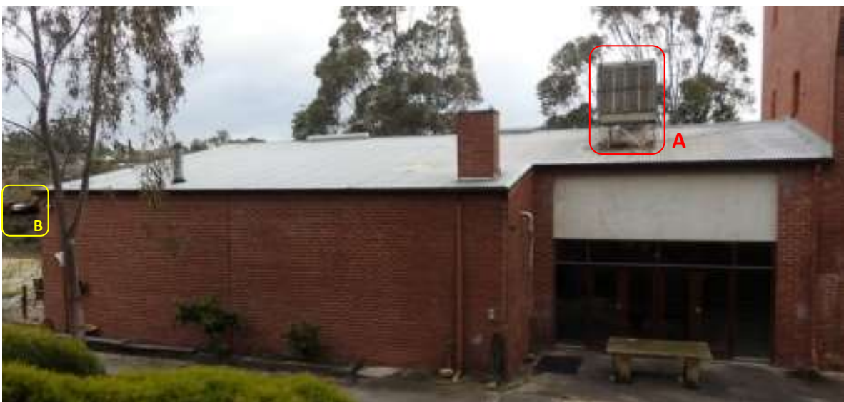
Figure 2. View of eastern wall (building extension)
