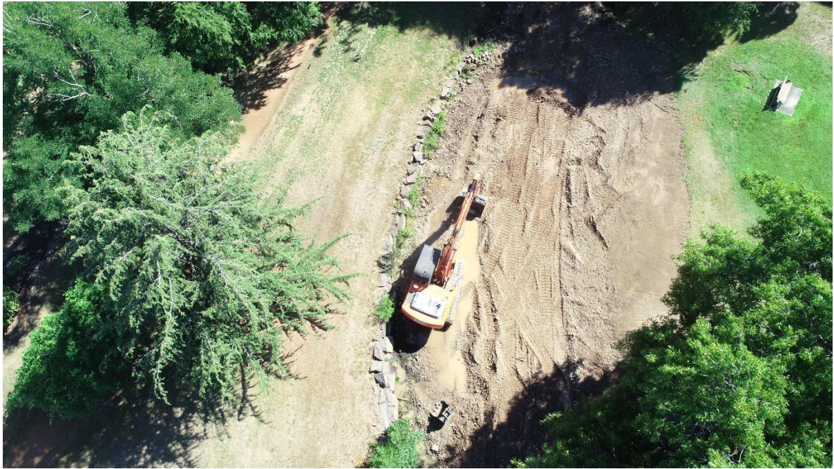
Repair works: Woody debris, sediment and gravel were cleared out of a section of UT Creek in Alexandra.
