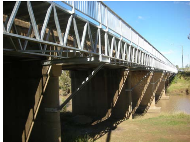
Above left: The construction of long bridges over the Goulburn River and several smaller creeks will be one of the major costs associated with the development of a trail between Alexandra, Thornton and Eildon. Above right: a 'clip on' bridge has been fixed to a road bridge in Surat, Queensland. A similar approach could be used for the two bridges across the Goulburn River.
