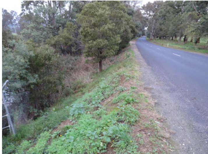
Not all sections of the preferred route are easy. Some steep sections along Back Eildon Rd will require a cantilevered boardwalk structure out over the steep embankment at the side of the road.
