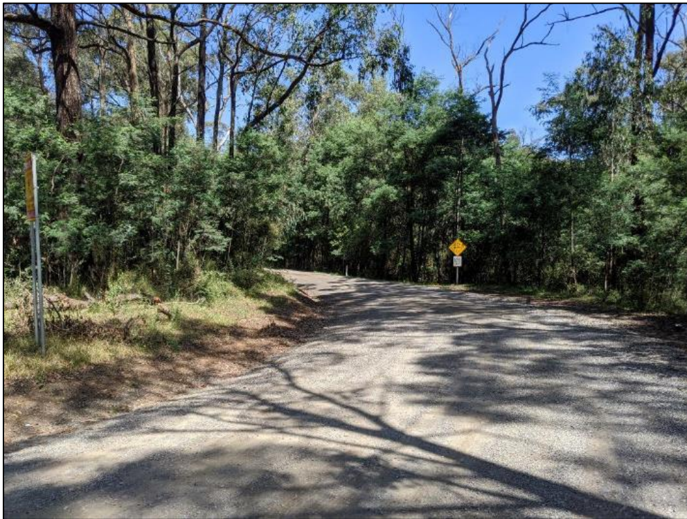
Photo 2: Gordons Bridge Road – Facing south-west
