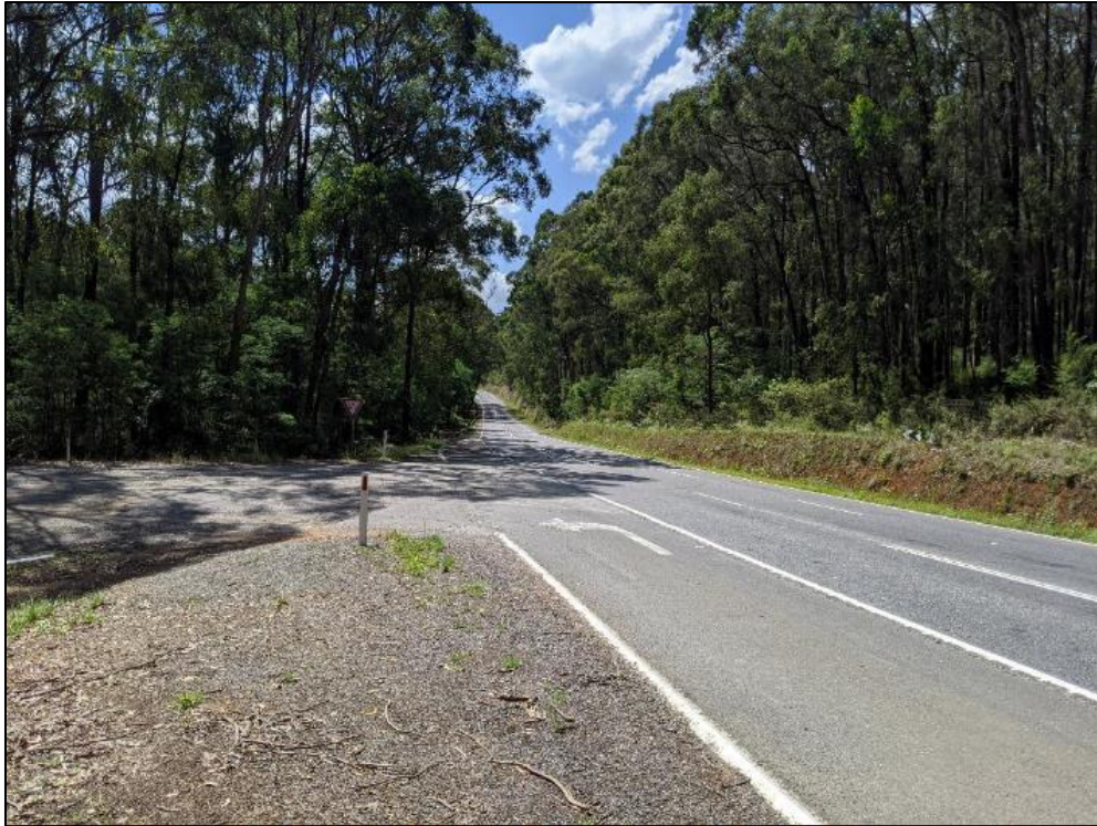
Photo 1: Intersection of Melba Hwy and Gordons Bridge Rd – Facing north
