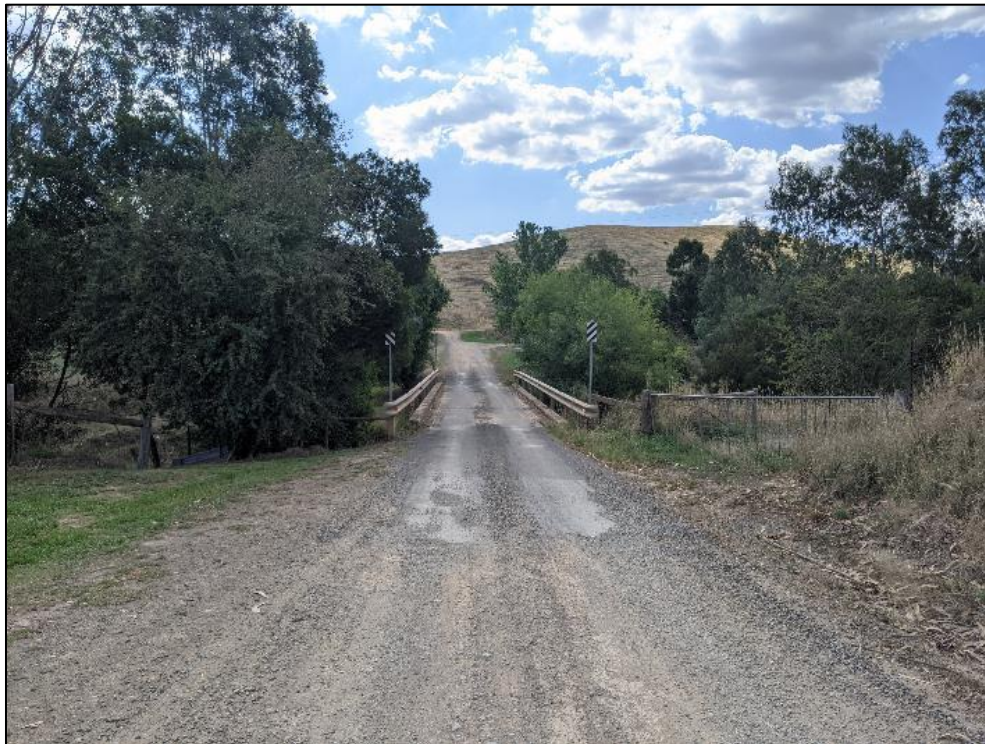
Photo 2: Johnsons Creek bridge – Facing north-west
