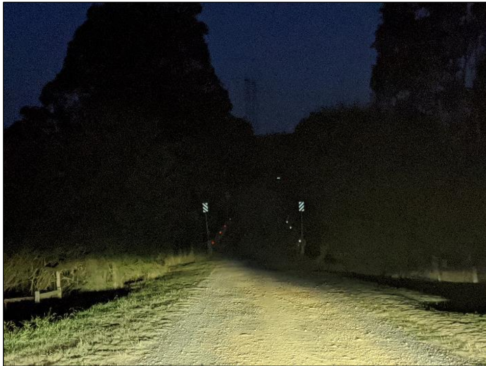
Photo 8: Johnson Creek bridge – Facing south-east (NIGHT)
