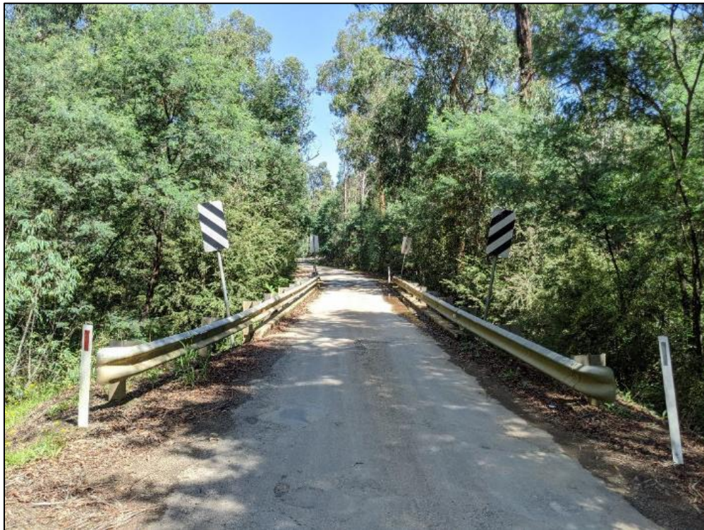
Photo 4: Bridge over Yea River – Facing south
