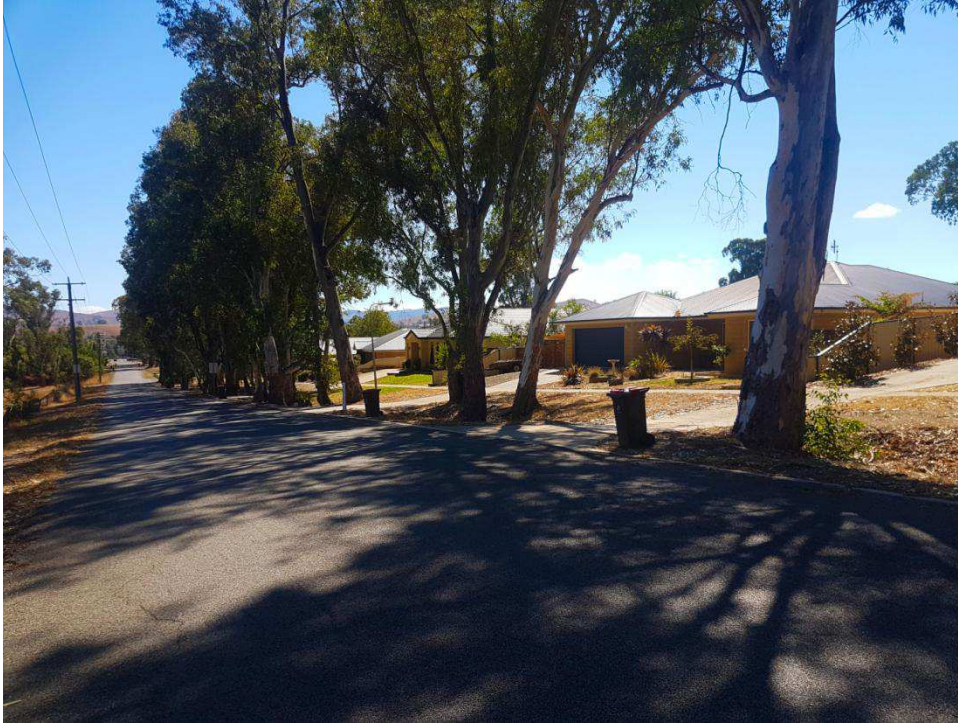
Photo 7: Facing south up Halls Flat Road showing cross-overs from previous developments to the north of the proposed development.
