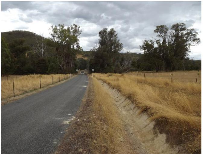
An open drain on Old Murrindindi Rd, susceptible to scouring, releasing sediment into Murrindindi River.
