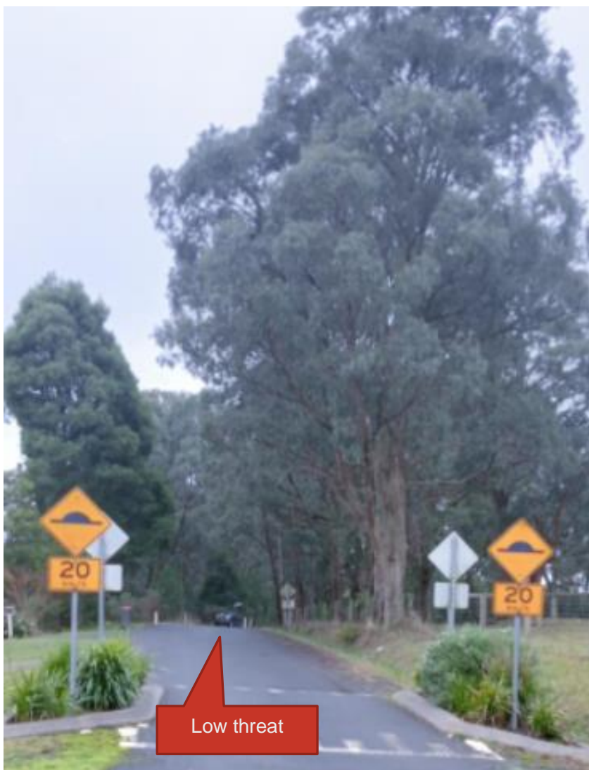
Photograph 9: The road reserve of Pratts Road is well managed and presents as Low Threat conditions
