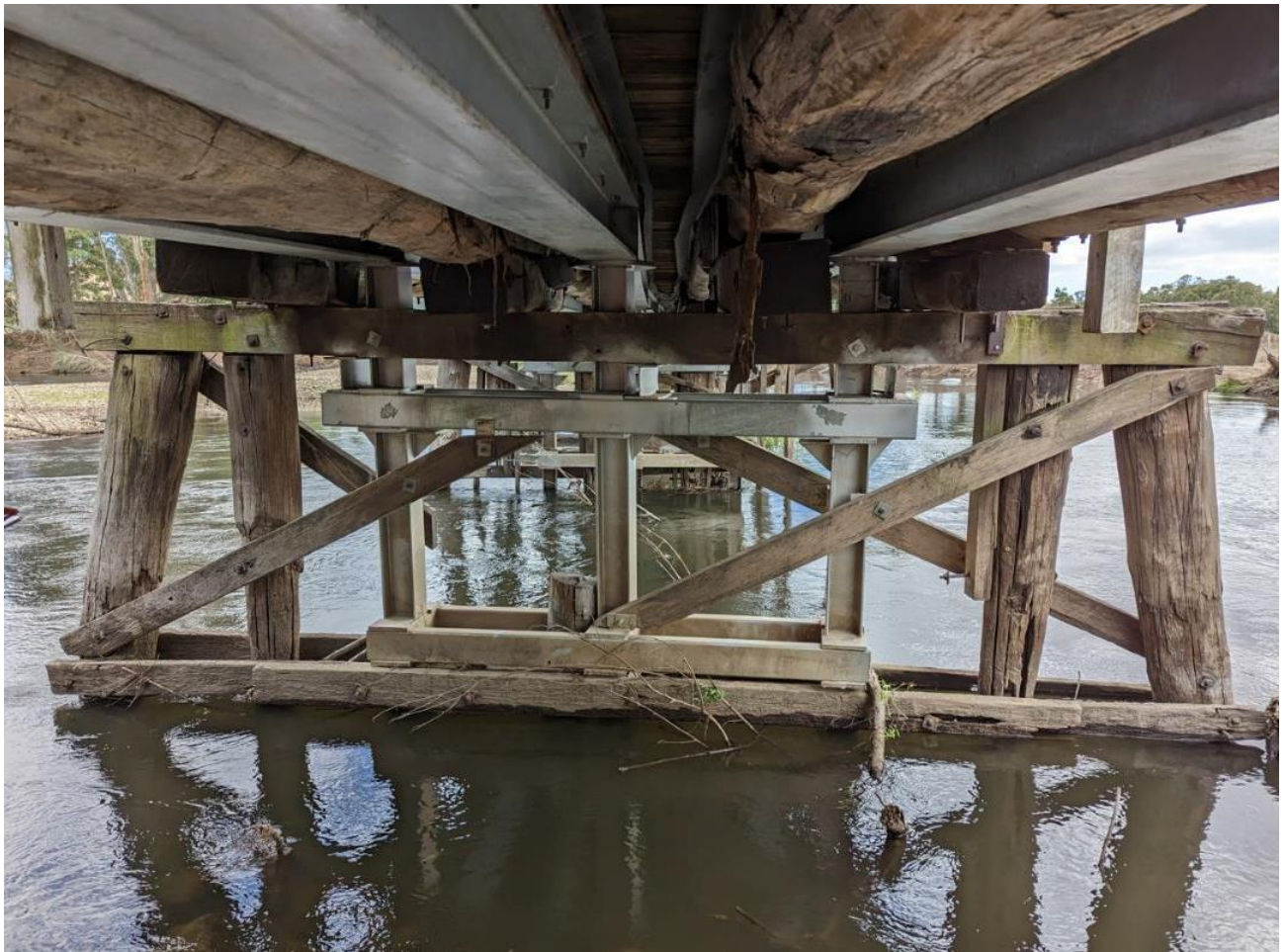
Photo showing the timber truss and steel frame beneath Breakaway Bridge
