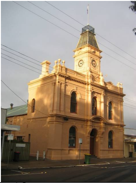
Yea Shire Hall Source: Context, 2008
