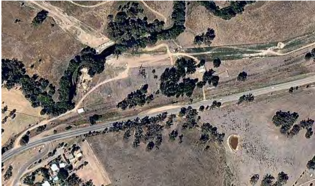
AP 1.1 Goulburn water pump station with white roof at left, shearing shed in middle
