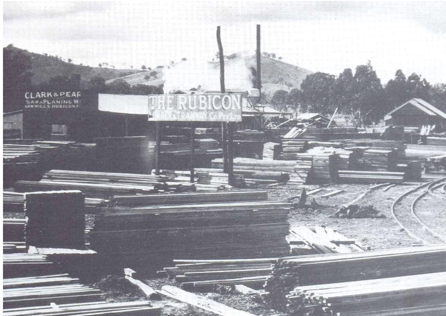
Figure 35 The Rubicon Lumber & Tramway Company's stacking yard at Alexandra
