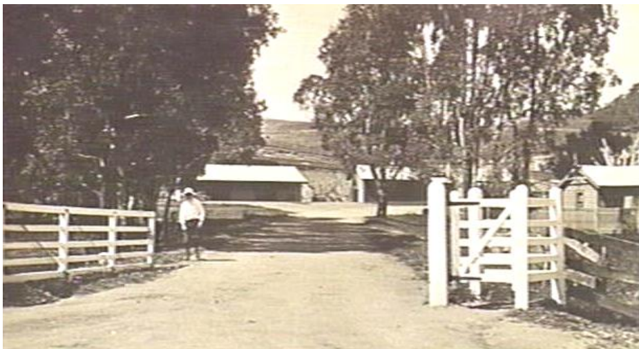
Figure 17 Entrance to Molesworth Railway Station, c.1914 Source: La Trobe Picture Collection, State Library of Victoria
