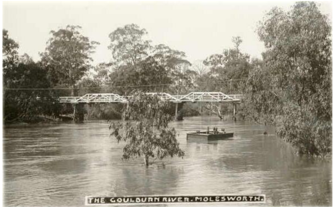
Figure 14 Bridge over the Goulburn at Molesworth, c.1912 Source: La Trobe Pictures Collection, State Library of Victoria
