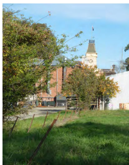
View of Shire hall building from Snodgrass St
