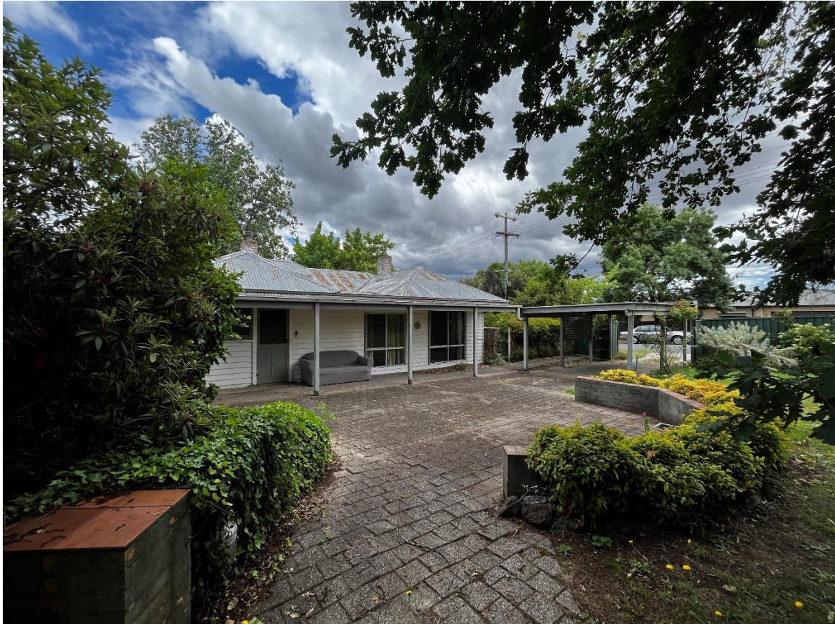
Figure 2.2: Existing dwelling and carport.
