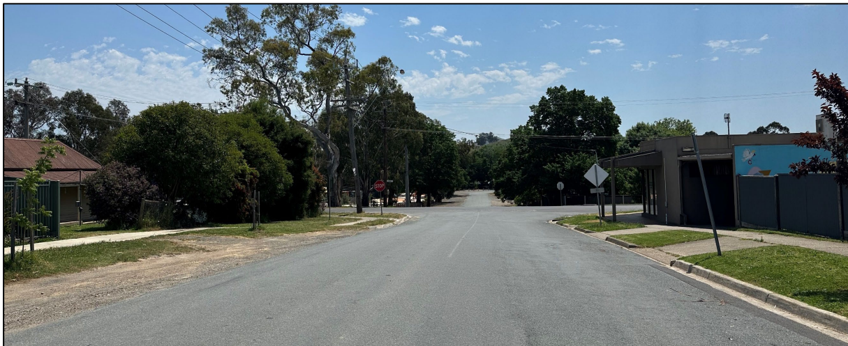
Figure 4: Bayley Street Looking North
