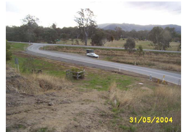
Photograph 6. There are problems with visibility, traffic movements and the location of the bus stop at the intersection of the Highway and Whanregarwen Road.
