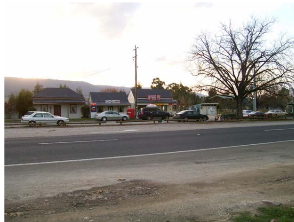
Photograph 4. The consistency of the built form within the main activity area is a key part of the town's character and heritage.
