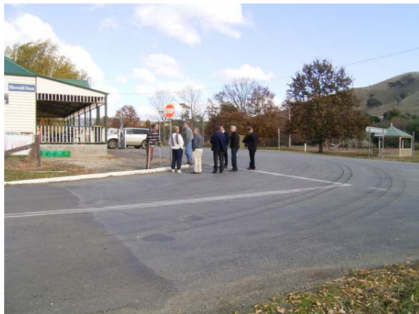
Photograph 2. The intersection of the Broadford-Flowerdale Road and King Parrot Creek Road – poor intersection layout requires improvement.
