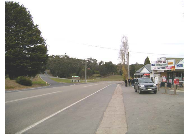
Photograph 5. Intersection of Maroondah Highway and Marysville Road. Dangerous turning movements in this area due to lack of visibility along the Highway.
