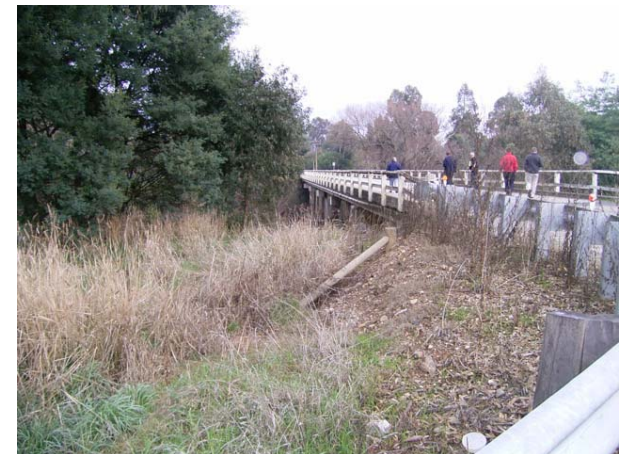
Photograph 6. The Back Eildon Road carries significant local and visitor traffic, however there is no means for pedestrians to safely cross the Goulburn River.
